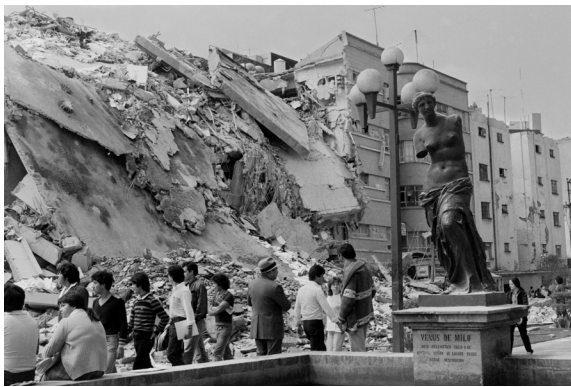
Buildings affected by the earthquake on the corners of avenues Alvaro Obregon and Insurgentes. September 19, 1985. © Elsa Medina
